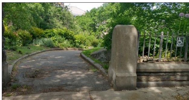
At Morningside Park in Manhattan, a designated wheelchair ramp was three times steeper than the allowable standard, had no handrails and was potholed. Source: State Comptroller
